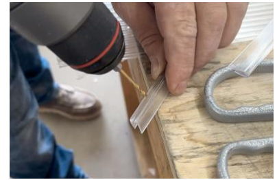
Attach U-Channel: Drill Weep Holes
