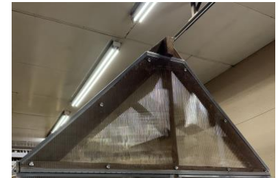
Side Roof Panel: Exterior View
