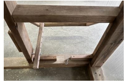
Front Window: Interior View
