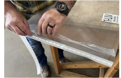
Edge Sealing: Anti-Dust Vent Tape
