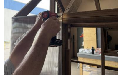
Front Wall Panels: Pre-drill Holes
